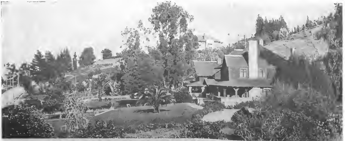
A Typical Bit of Pasadena, Cal.—In the Foreground Are the Homes of Two Directors of the Petrolithic Movement.
